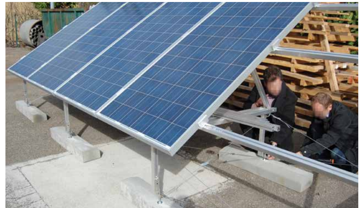
Solar Panel Installation
